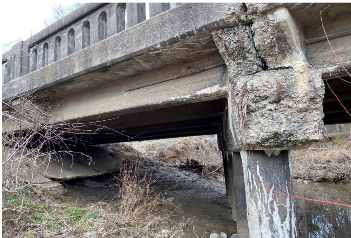
2 - IMG_2758 Bridge Below Deck - Facing N.JPG
