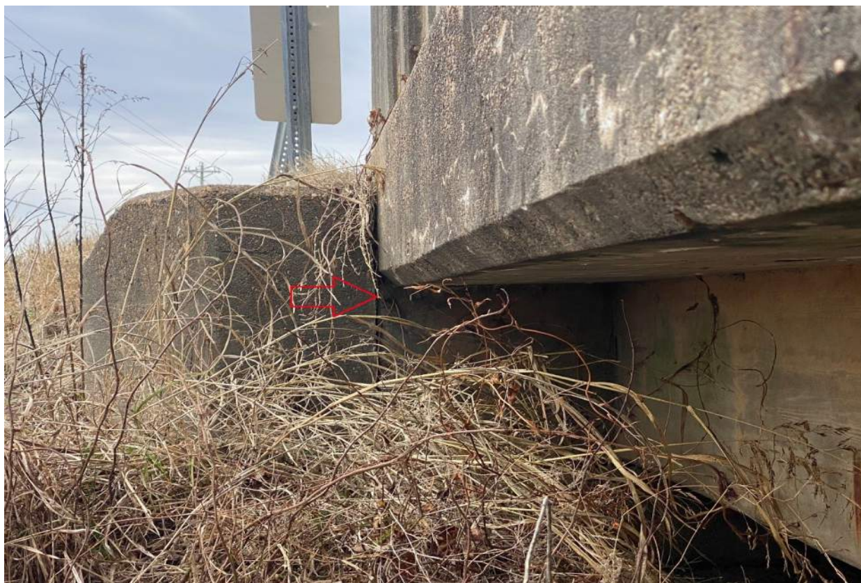
4 - IMG_2760 Abutment Joint - Facing W - Sample I-10116-1.JPG
