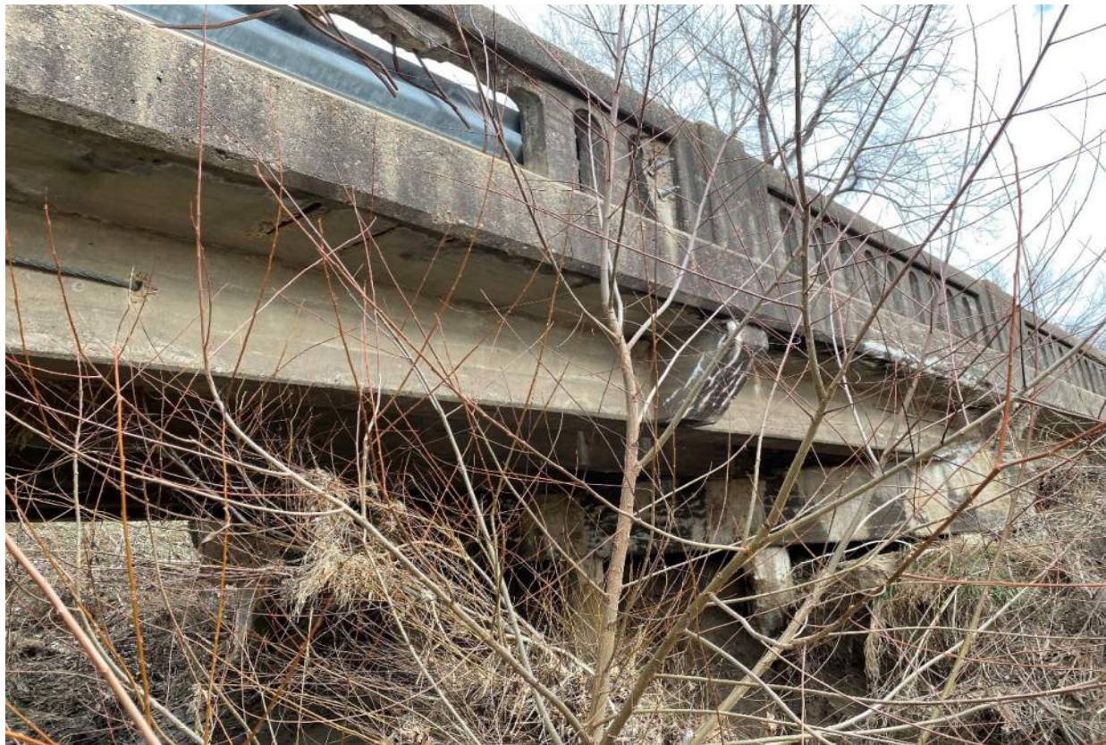
3 - IMG_2759 Bridge Below Deck - Facing E.JPG
