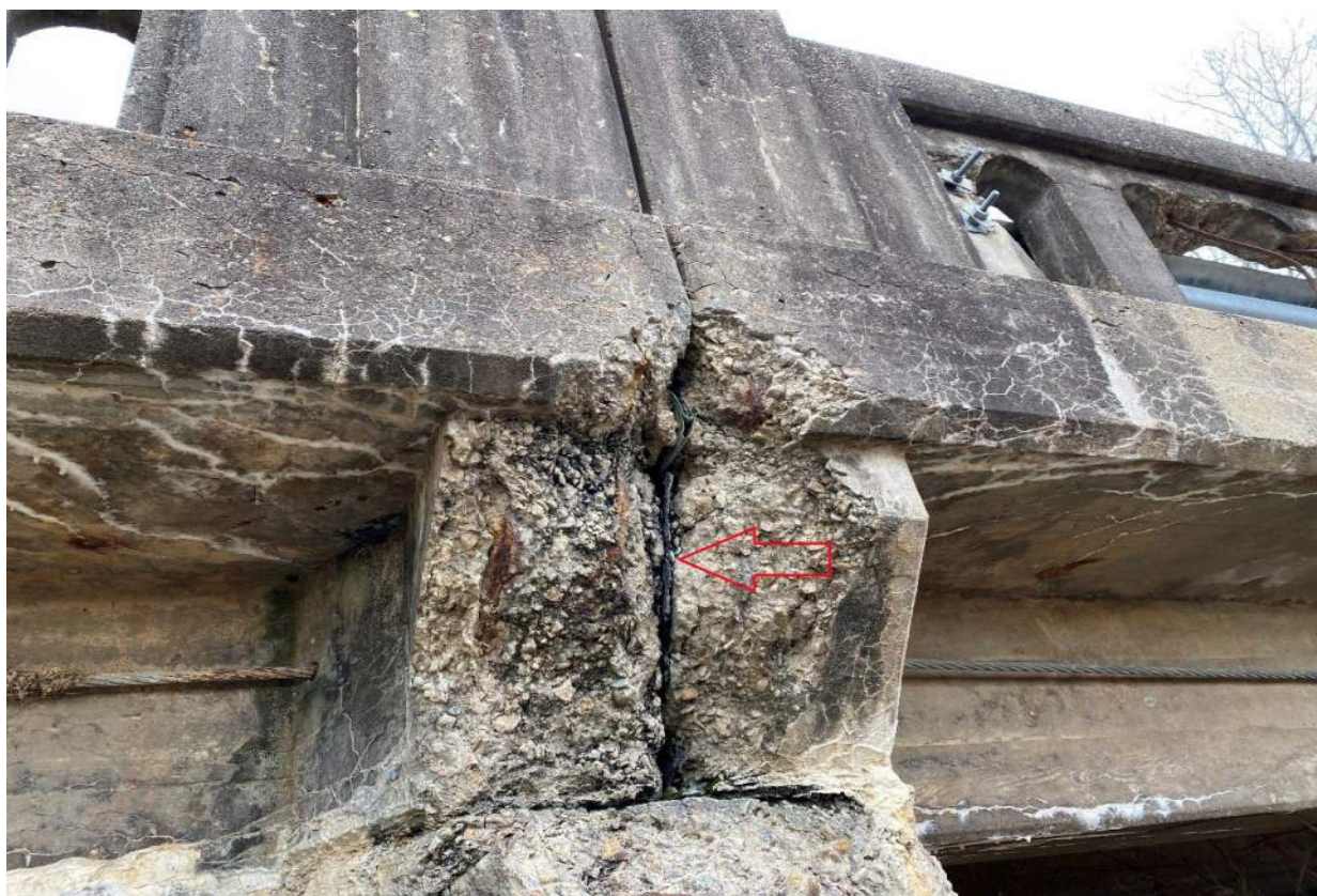
6 - IMG_2762 Vertical Joint in Deck and Girder - Facing N - Sample I-10116-3.JPG
