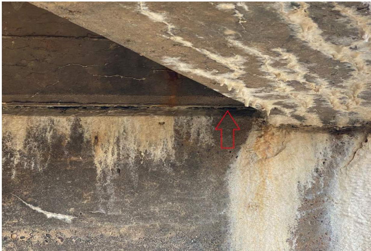
5 - IMG_2761 Joint at Pier Cap - Facing E - Sample I-10116-2.JPG
