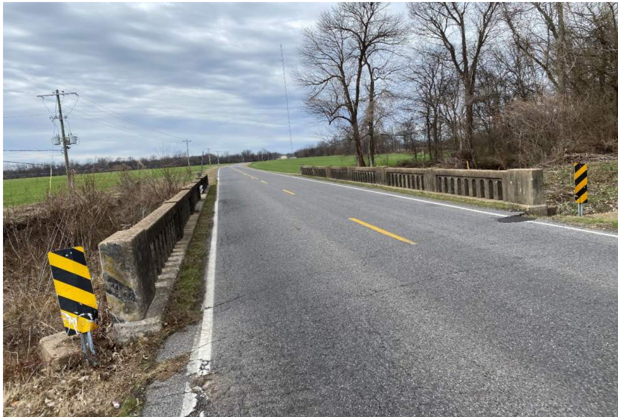
1 - IMG_2757 Bridge Surface - Facing W.JPG
